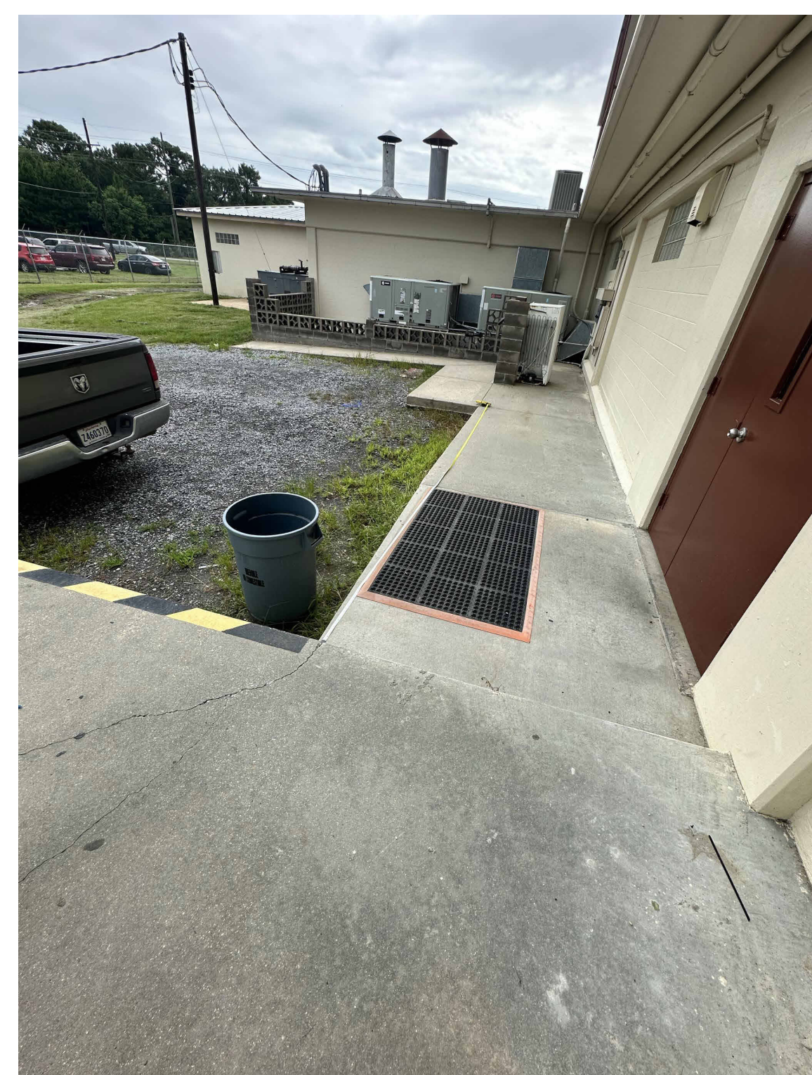
EXISTING SLAB CONDITION NORTH @ 1ST FLOOR - CENTER N.T.S. 7
