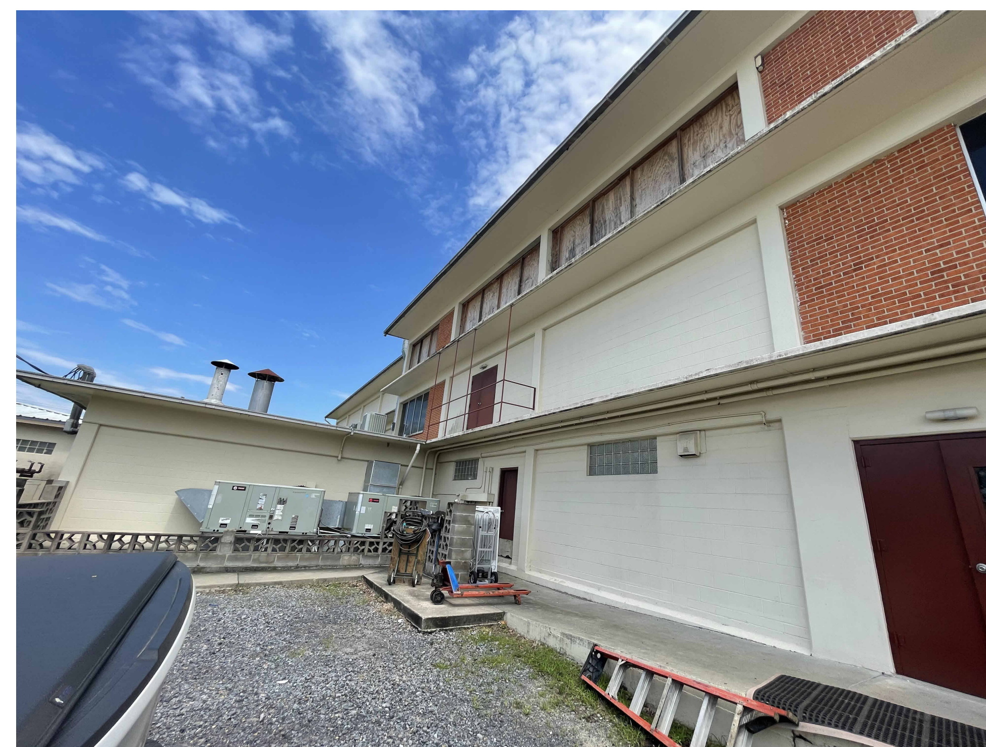
EXISTING NORTH FACADE - MECHANICAL N.T.S. 4
