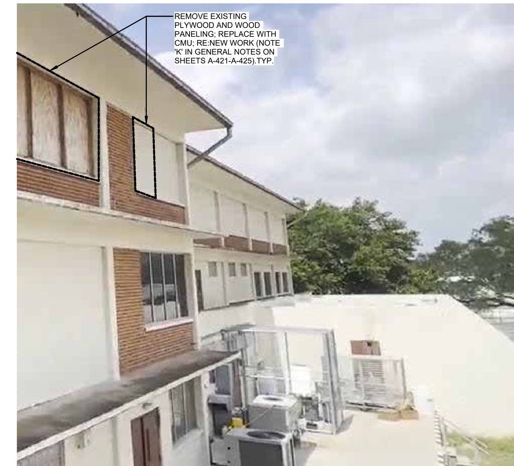
EXISTING NORTH FACADE - WEST WING N.T.S. 2
