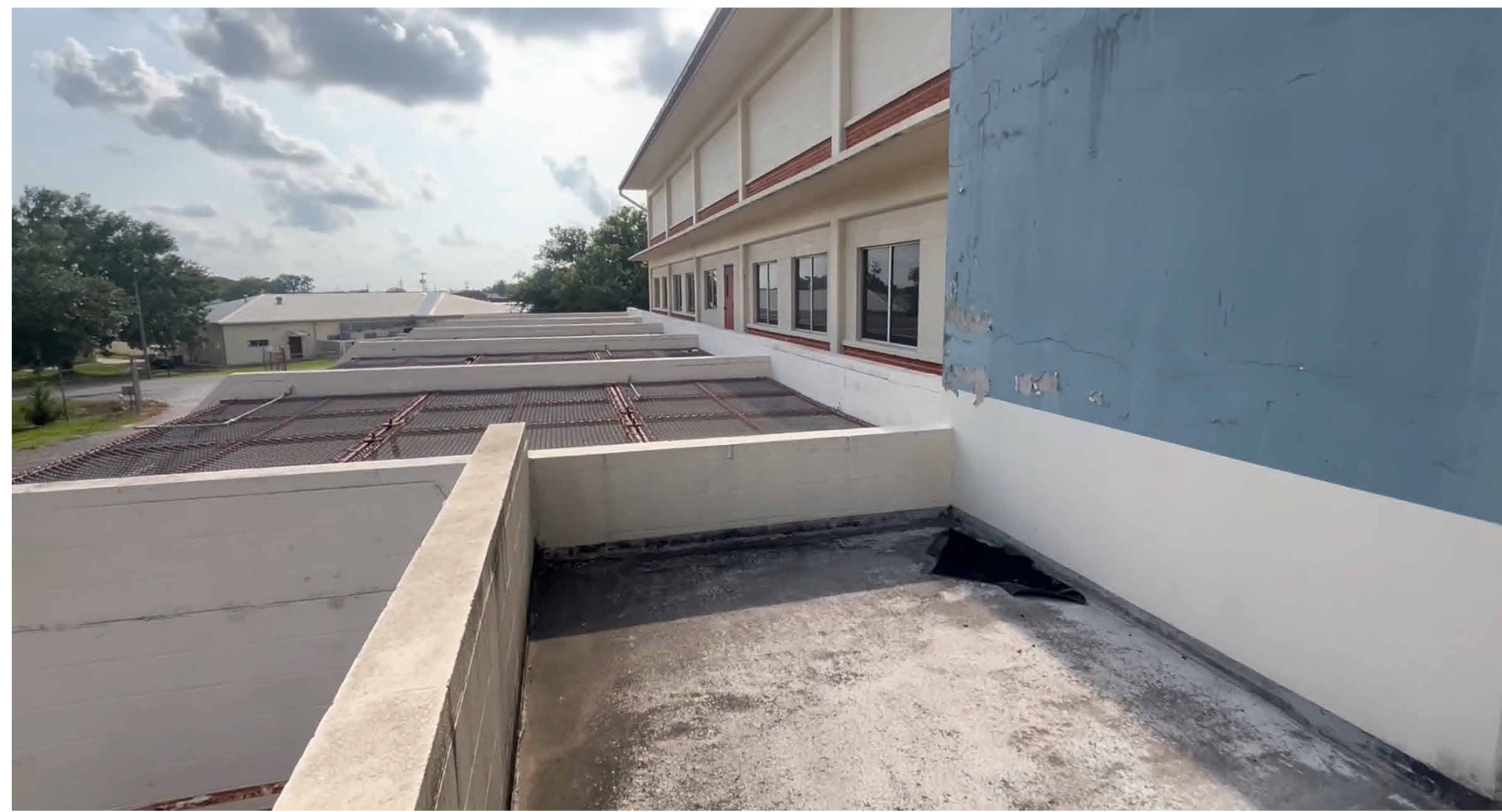
EXISTING SOUTH FACADE - WEST WING N.T.S. 9
